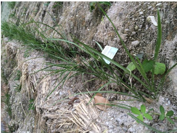
Figure No. 5. Soiltraps working at cut slope. Kindly by Vetiver tec. Guatemala.
