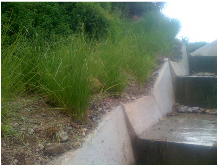
Figure No 2. Structure to reduce hydraulic energy. Kindly by Vetiver tec, Guaemala.
