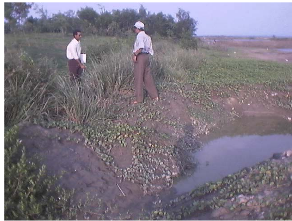
Fig 3: Vetiver planted at the seaside toe line.
