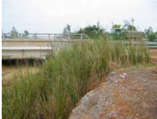
Photo 11: A well-stabilised bridge abutment on Highway 1 in Quang Binh province
