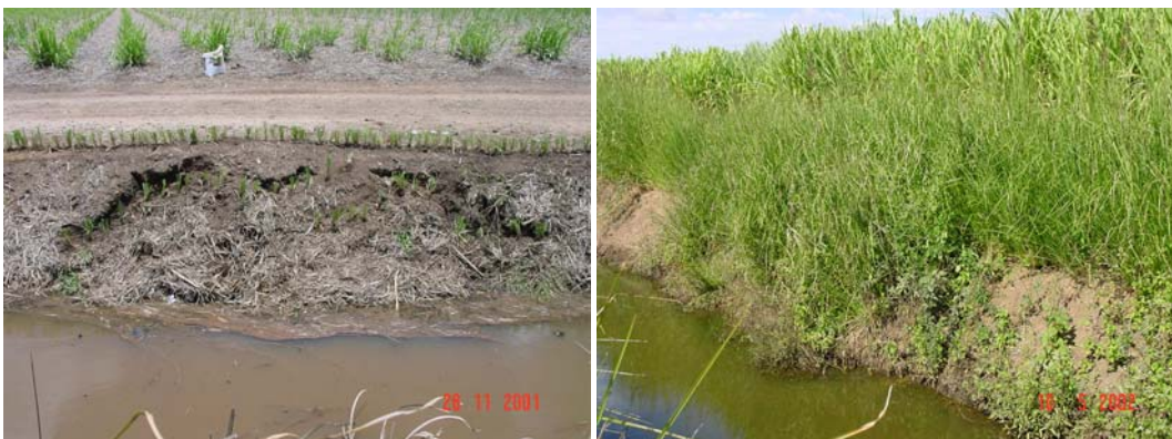
Photo 3: Vetiver was planted on this eroded section in November 2001 (left) and it was completely stabilised 6 months later (right).
