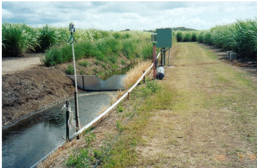
Photo1: Multipoint Sensor Chamber mounted in electronics cabinet, pluviometer, pressure transducers, runoff and vetiver planted section weirs.
