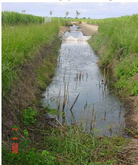
Photo 5: Establishment of other plants provided further protection to the steep and highly erodible slopes
