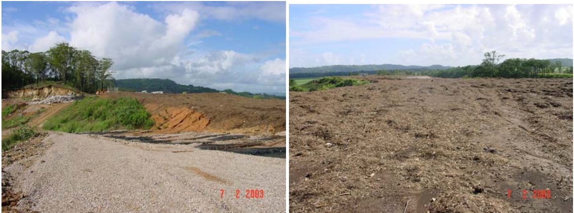
Photo 6: Side view (left) and top view (right) of the landfill mound, which has been mulched.
