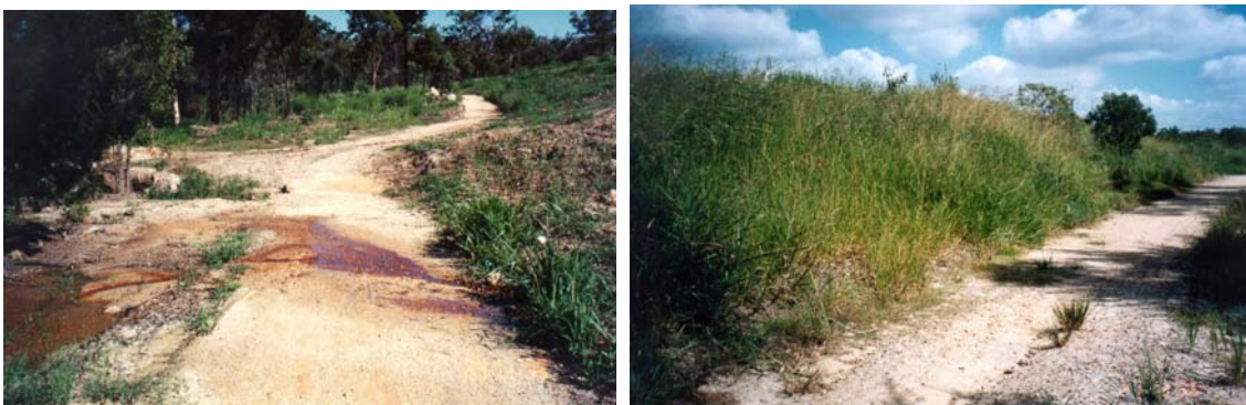
Photo 4: Left , Toxic leachate seepage at the foot of an old landfill at Cleveland Right , One year after planting, Vetiver grew well and dry up the seepage
